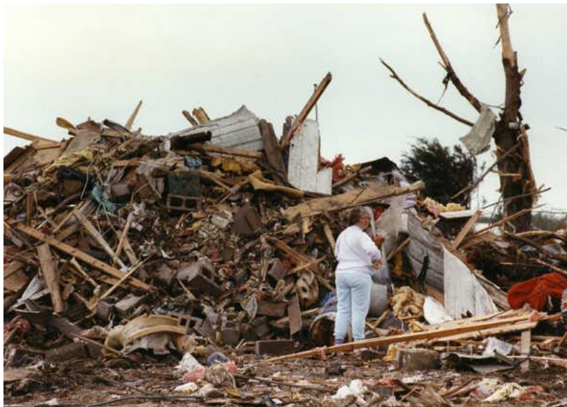
Figure 11: 113 The Golden Spur Mobile Home Park was almost completely destroyed in the April 1991 tornado. (reprinted with permission of the Wichita Eagle)
