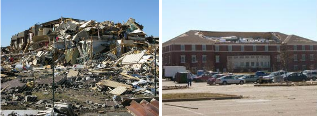
Figure 12: 120 The picture of the left shows the complete destruction of the wood frame Jelks dormitory, whilst the masonry academic building, Jennings hall (right) experienced damage only to the roof. (Source: AIR Worldwide)
