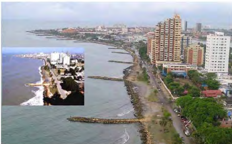
Figure 16-2 – Beach protection measures along Bocagrande. Source: Invemar, 2005
