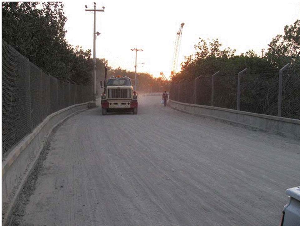
Figure 5-13 – Road between the mainland and Isla del Diablo
