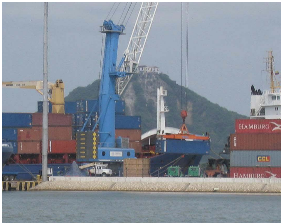
Figure 7-2 – View of MEB, including a drainage outlet into the sea
