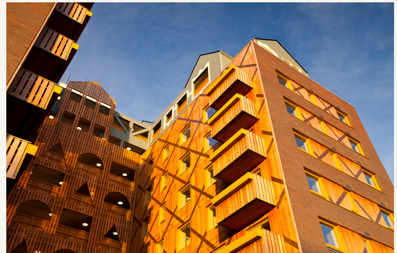
Riverside One, in Teeside, UK, is an exceptional green building whose individual housing units have a low carbon footprint. The whole block is heated by a biofuel boiler. During construction it used recycled oil rig pipes for piling, the concrete was mixed with recycled aggregate, super insulated with earth wool, it uses grey recycled water to save water, locally sourced timber, the electricity for the building is sourced from renewable sources and the building incorporates Swift bird boxes and bat boxes. © Global Warming Images / WWF
