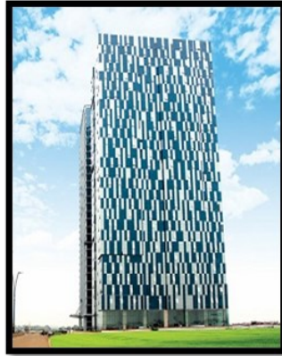
GIFT Two Tower Basement + 28 floors 0.8 Mn Sq. Ft BUA (DTA) Tallest Tower in Gujarat
