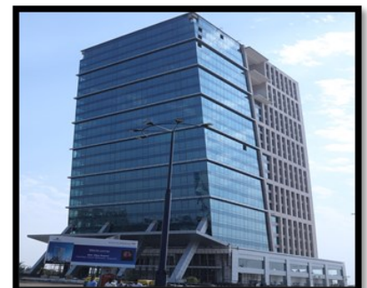
PRAGYA TOWER (SEZ- IFSC) 24 Storey - 0.5 Mn Sq. Ft BUA
