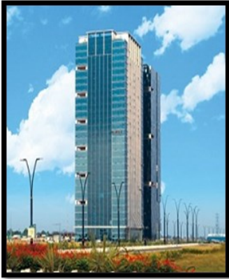
GIFT One Tower Basement + 28 floors 0.8 Mn Sq. Ft BUA (DTA) Tallest Tower in Gujarat
