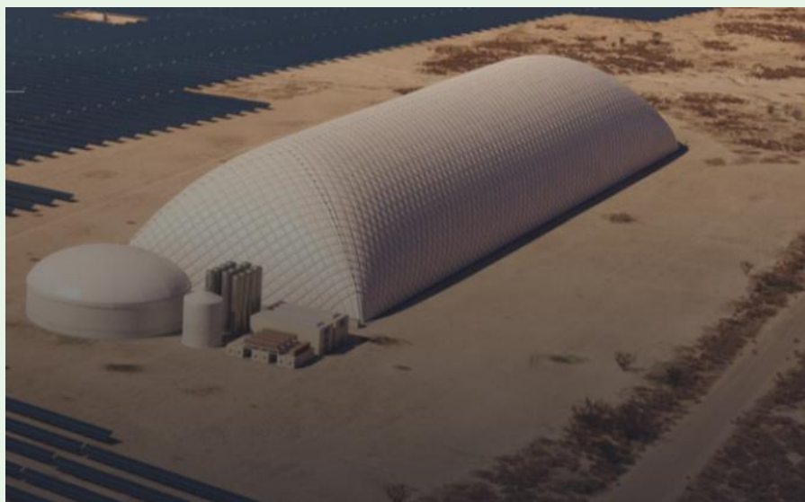
EnergyDome CO 2 Battery, Sardinia
