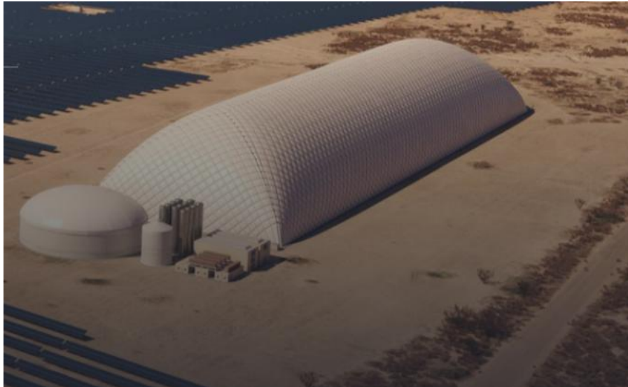
EnergyDome CO 2 Battery, Sardinia
