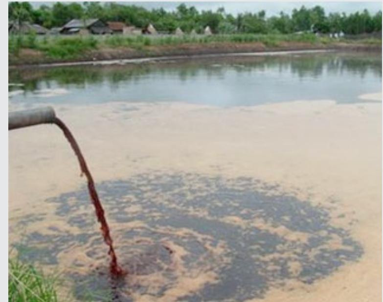
A pipe releases untreated wastewater from the Vedan plant into the Thi Vai River in Dong Nai Province
